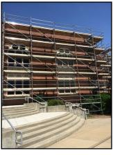
We expect that the sealant will be applied to the upper portions this week and then it is on to the remaining east wall. We have intentionally focused on the upper portions so as to negate, as quickly as possible, the rental cost of the scaffolding. The lower 20' or so will be repointed later using our contractor's own scaffolding.
