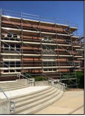
Work on Phase 1 (the 1950s building) of the exterior repairs is about 50% complete now. The windows have been re-caulked and painted, gutters have been repaired and a sampling of sub-roofing has been inspected (and found to be sound). Power washing will begin next week and, once dry, a sealant will be applied. We anticipate the movement of scaffolding to the Phase 2 (east side of the 1920s building) section to begin towards
